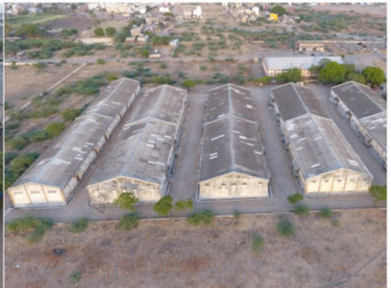
WAREHOUSE, WAKHAR MAHAMANDAL (JADHAVWADI)
