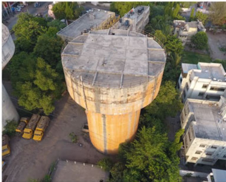
ELEVATED WATER STORAGE RESERVOIR (CIDCO)
